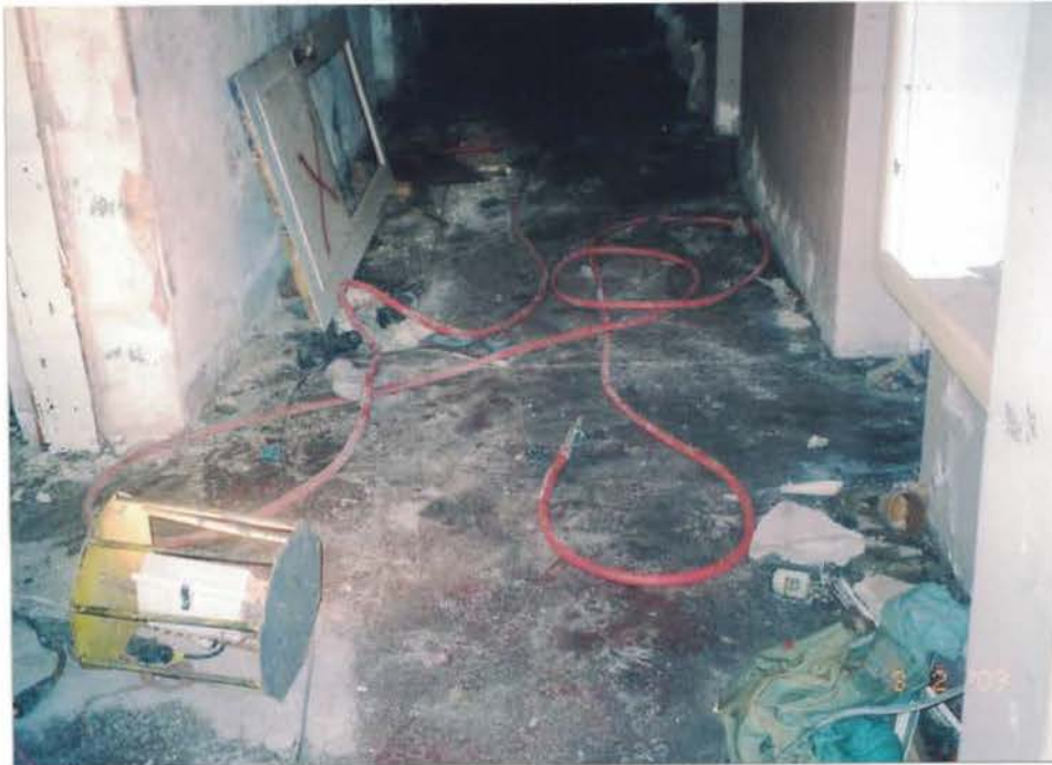
Photo #13: Spray used wet methods to remove LBP doors for off-site stripping of LBP. Water sprayed on the components minimized leaded dust, mold spores, and mouse allergens from becoming aerosolized during the cleanup activities. Viewing down, and to the north inside the basement.
