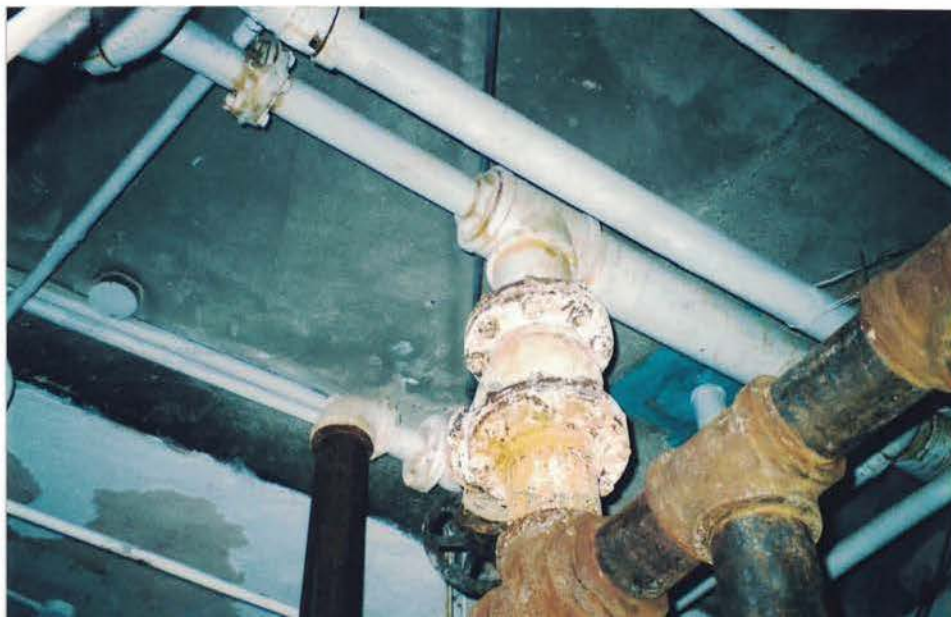
Photo #33: TSI boiler insulation was removed from the hot water tank, and TSI pipe insulation was removed from the pipes. Note that turquoise duct tape was used to cover open ends of pipes to prevent potential contamination from asbestos fibers. Viewing southwest.
