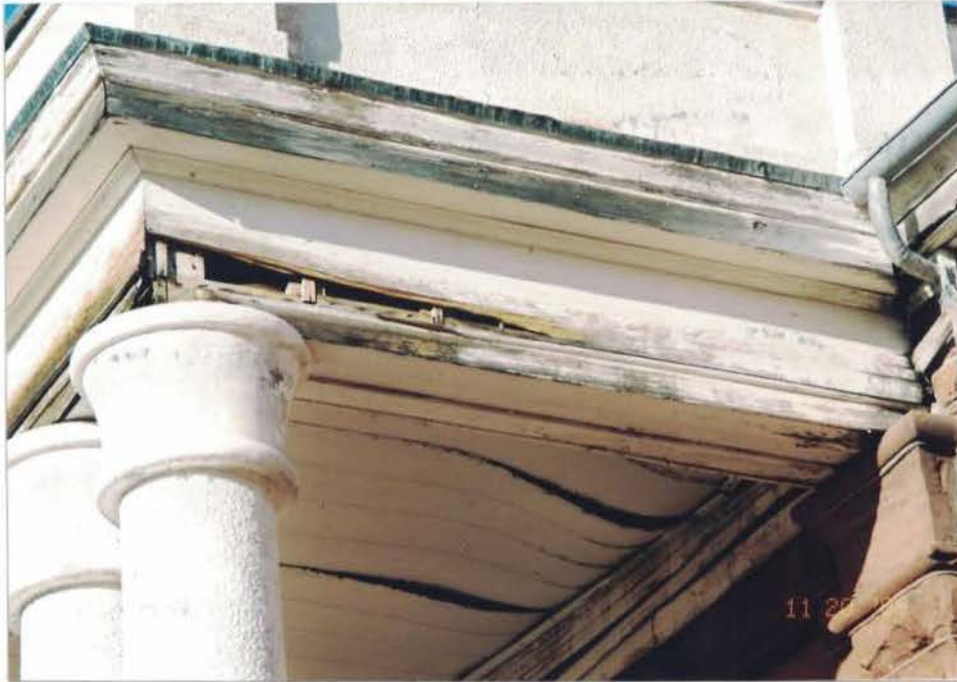
Photo #5: Water-damage on the portico roof has resulted in buckling of the wooden ceiling, and deterioration of structural components. The portico roof drains eastward toward the main roof, and is not equipped with scuppers or gutters. Viewing up, and to the northeast.
