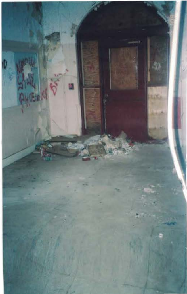
Photo #13: Spray used wet methods to remove LBP doors for off-site stripping of LBP. Water sprayed on the components minimized leaded dust, mold spores, and mouse allergens from becoming aerosolized during the cleanup activities. Viewing down, and to the north inside the basement.
