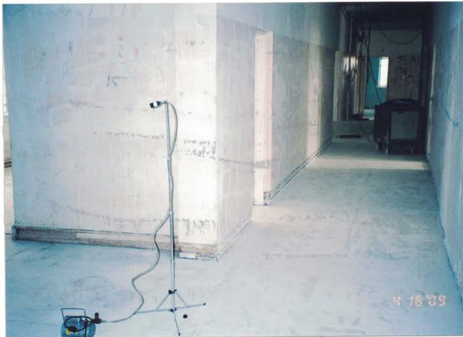
Photo #49: Post-abatement air sample 09TEC104-19, collected in the central portion of the 1st floor near the main entry, is reported with an airborne count of < 17 str/mm 2 of asbestos which is well below the AHERA clearance standard of < 70 str/mm 2 . Note the thorough layer of encapsulant on the concrete floor following the removal of asbestos-containing vinyl floor tile and black mastic. Viewing northwest.
