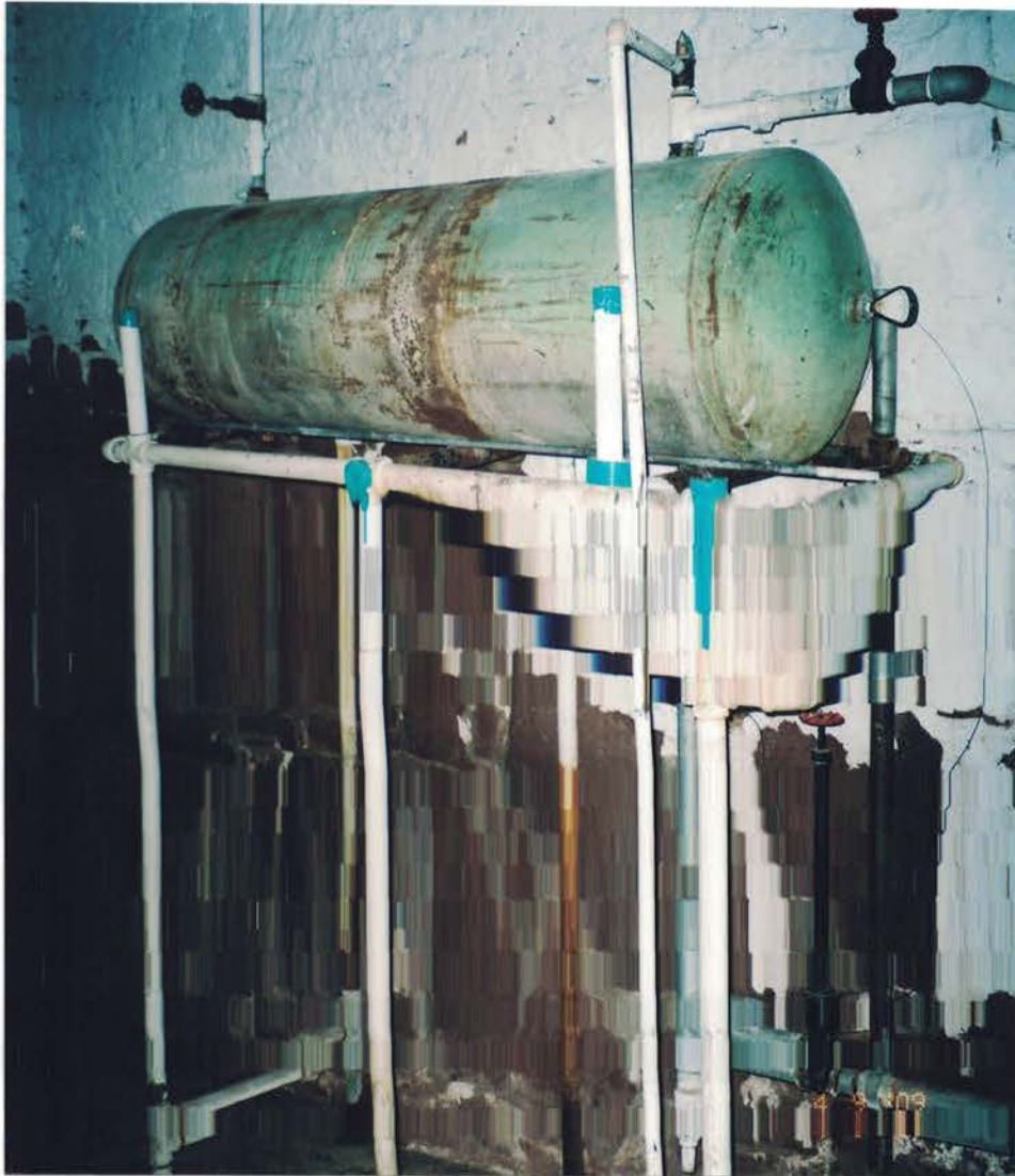
Photo #33: TSI boiler insulation was removed from the hot water tank, and TSI pipe insulation was removed from the pipes. Note that turquoise duct tape was used to cover open ends of pipes to prevent potential contamination from asbestos fibers. Viewing southwest.
