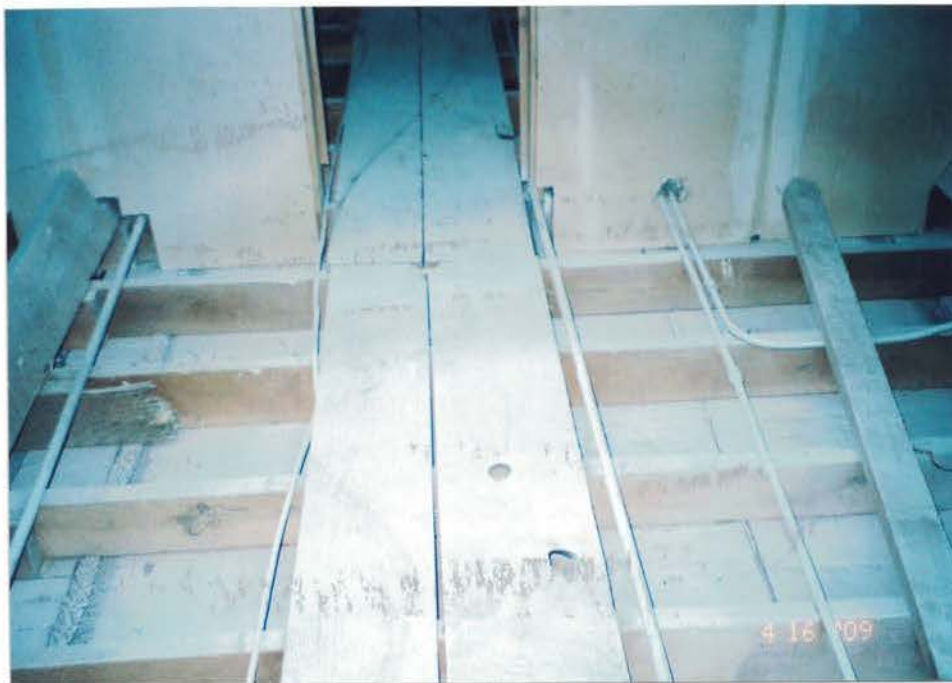
Photo #42: Inside the attic, rodent droppings, bat guano, fiberglass insulation, and building materials were thoroughly removed. Spray used Quat 128 and bleach to bioclean the wall and floor systems inside the attic prior to the application of a light layer of encapsulant. Viewing down, and to the north.
