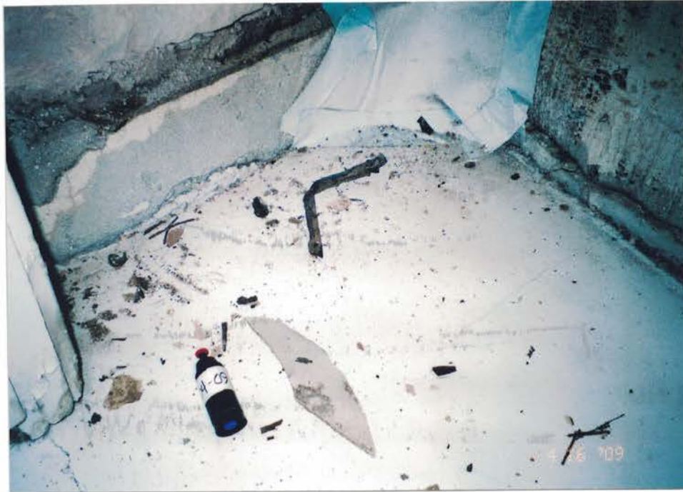
Photo #45: Post-remediation dust sample 09TEC104-09, collected from the 2nd floor Room 2-8 northwest closet, is reported with < 0.039 micrograms per gram (mg/g) of mouse allergens which is well below the threshold value of 1.6 mg/g. Based on the visual, Tallpines requested that Spray reclean the closet. Viewing down, and to the northwest.
